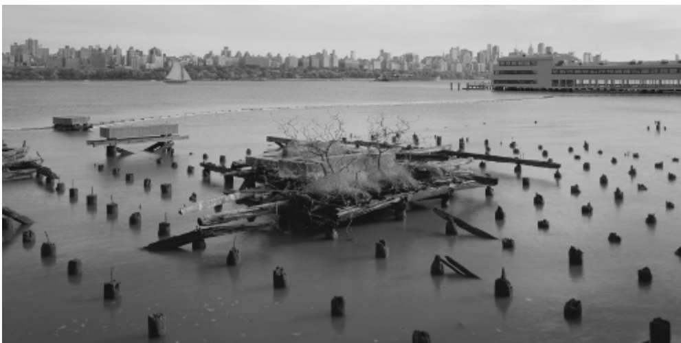
Figure 7.3 Quanta Resources Superfund Site, Bergen County, NJ (day 1 of Superfund365 ).
